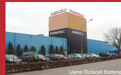
Usine Duracell Batteries
